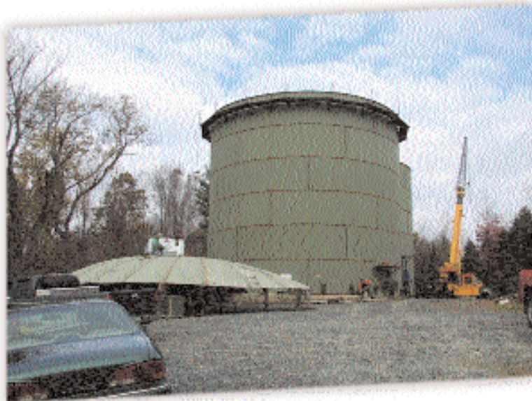
KJ's two water tanks (when under construction), which aid the groundwater wells in dealing with peak and off-peak demand.
